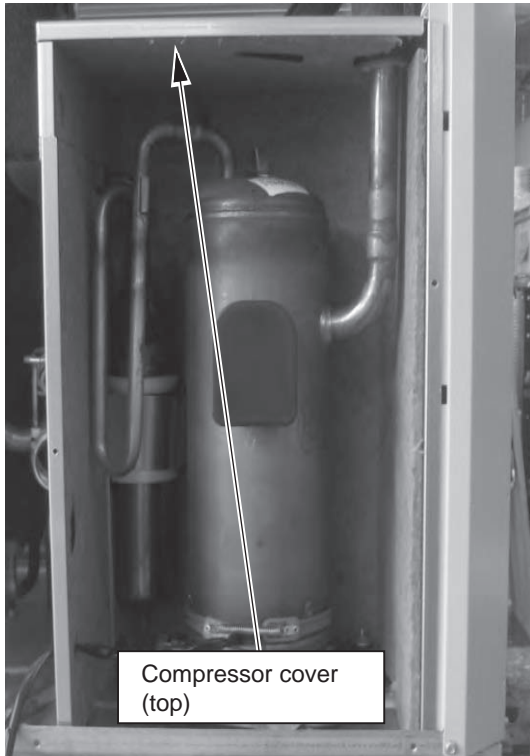
4. Remove the compressor cover (top).
